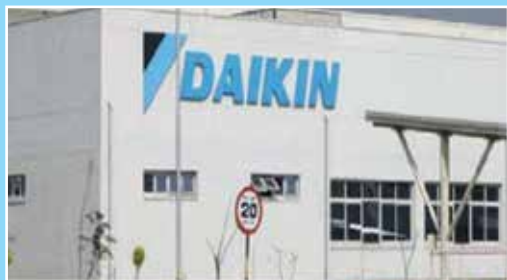
Daikin Air-Conditioners (Neemrana)
